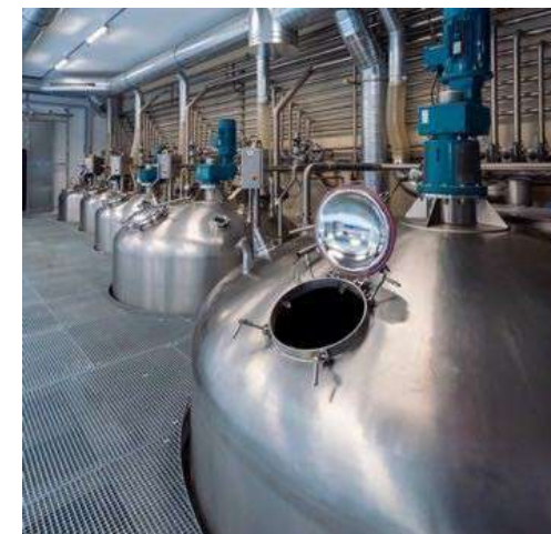
Mixing tanks - 3m 3 , 3m 3 , 6m 3 , 10 m 3 , 32 m 3
